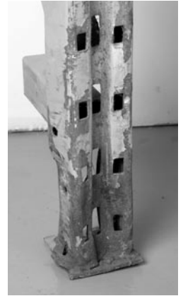
Corroded steel column worn by friction and rewelded (Photo: Maurice Vézinnet)
