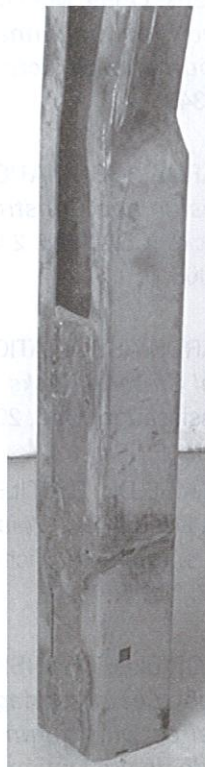
Figure 57. Damaged column repaired by electrode welding (Photo: Maurice Vézinnet)
